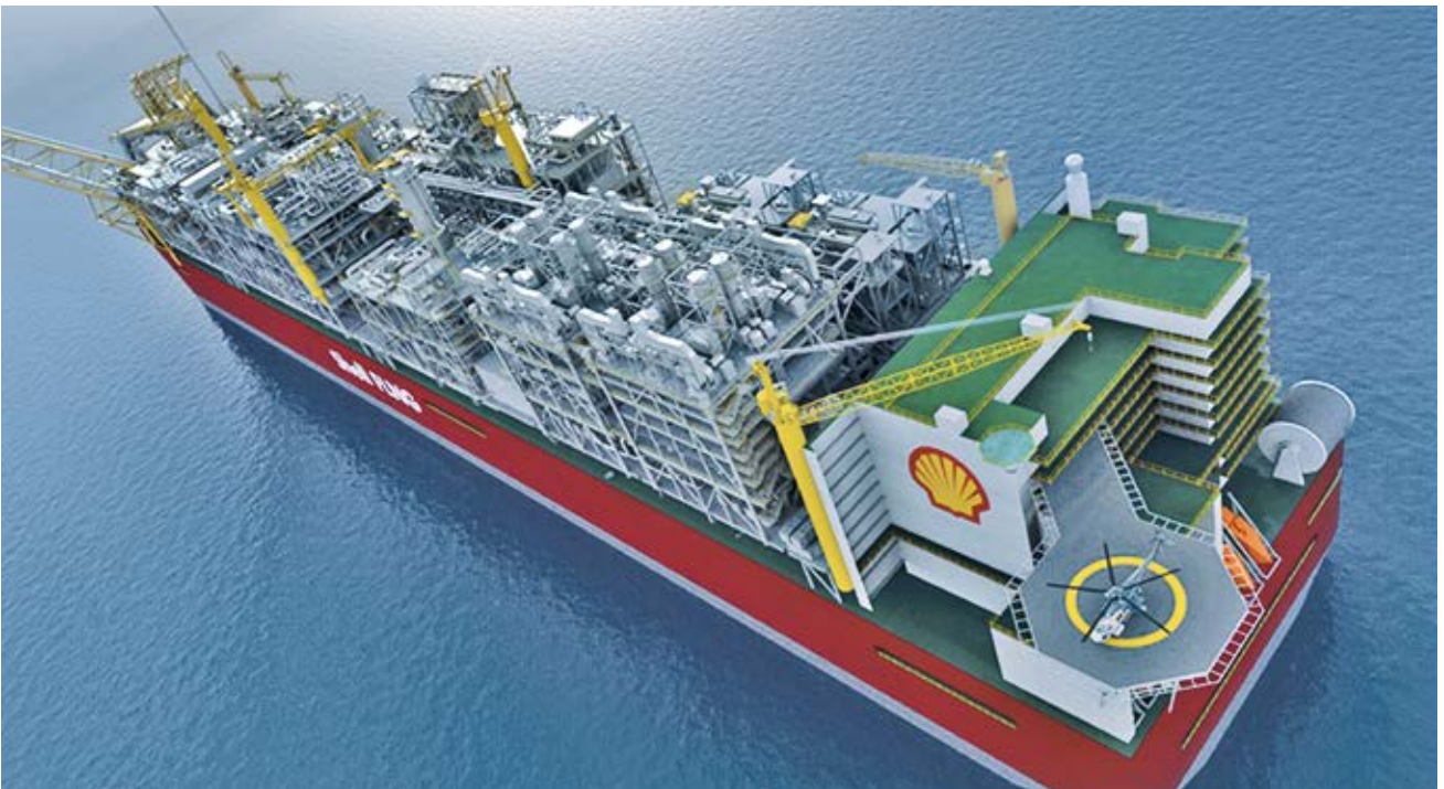
The largest FPSO in the world for natural gas production and liquefaction under construction – with 11 GEAFOL ADFW transformers of 6,300 to 20,000 kVA
